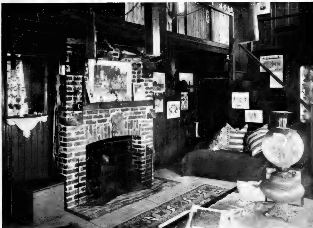
9—The Living-Room is Open to the Roof and is Finished in Dark Wood
